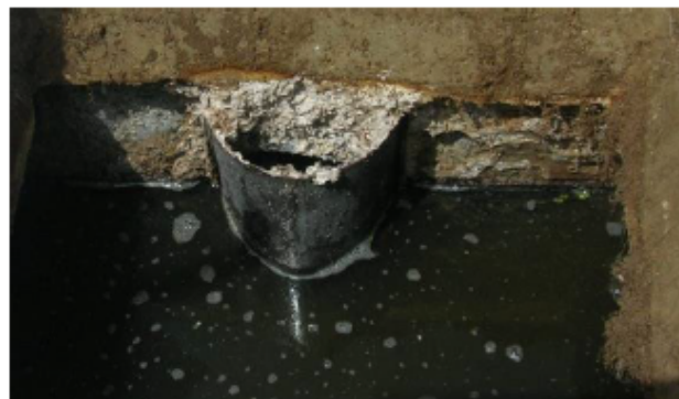
Photo 1 Concrete Corrosion around Outlet Baffle
