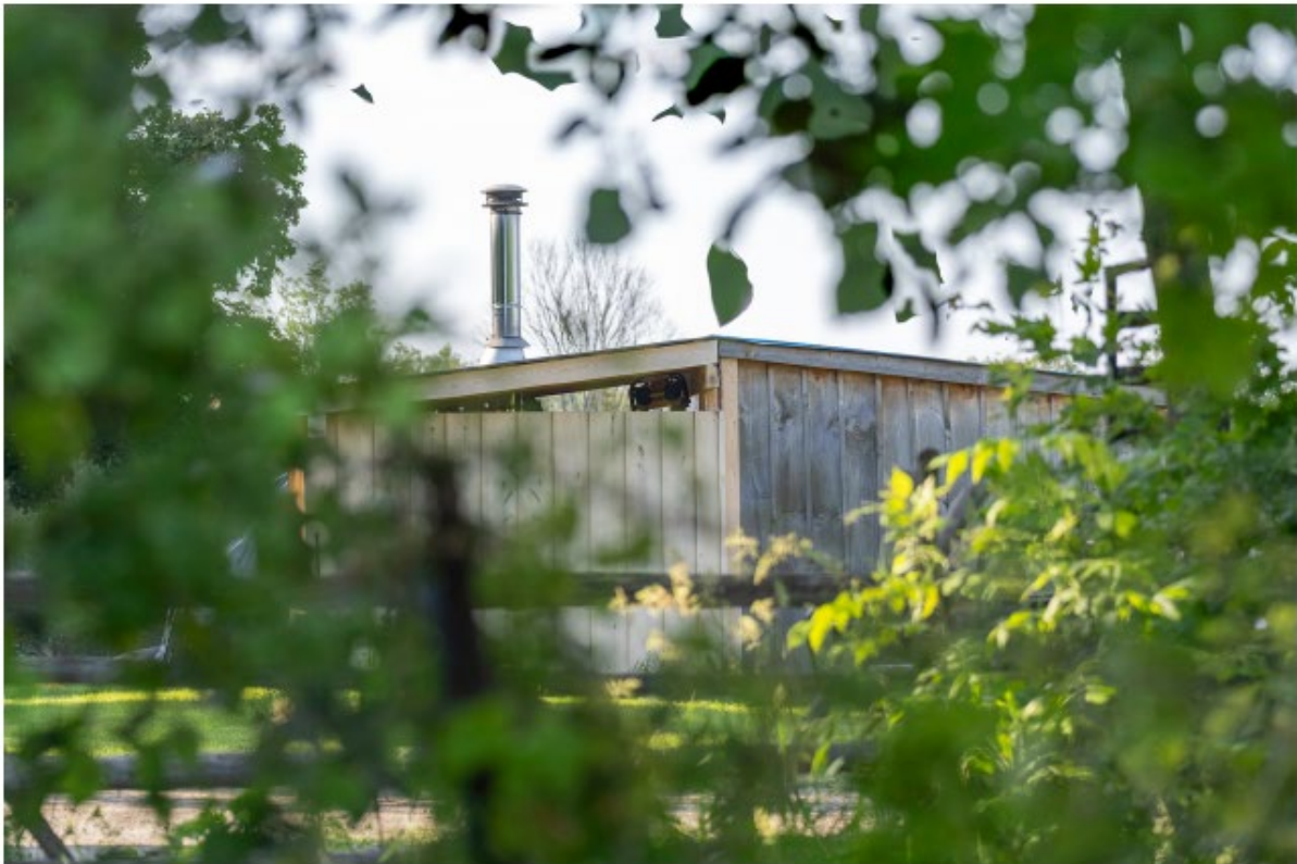
Figure 1: The wood furnace's shed
