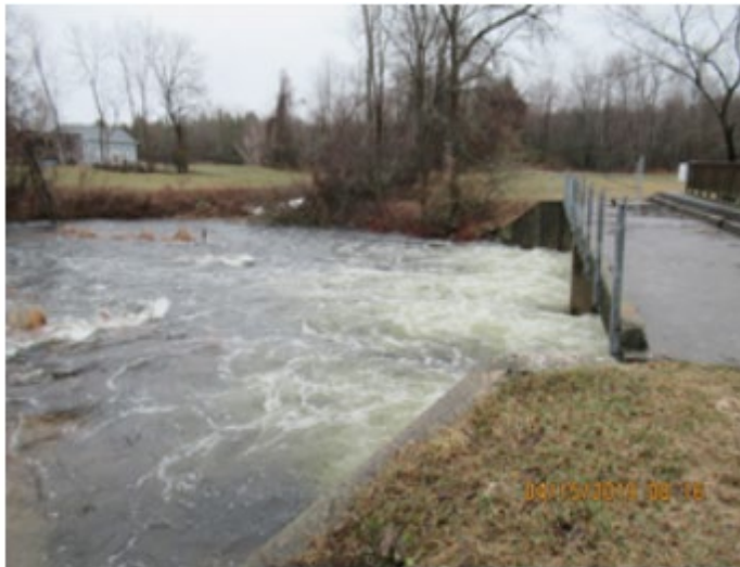
Photo 55 Downstream View of Bennett Dam
