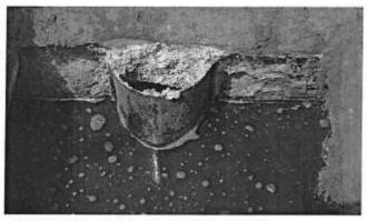
Illustration 1: Concrete Corrosion around Outlet Baffle
