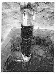
Illustration 2 - Clogged Effluent Filter
