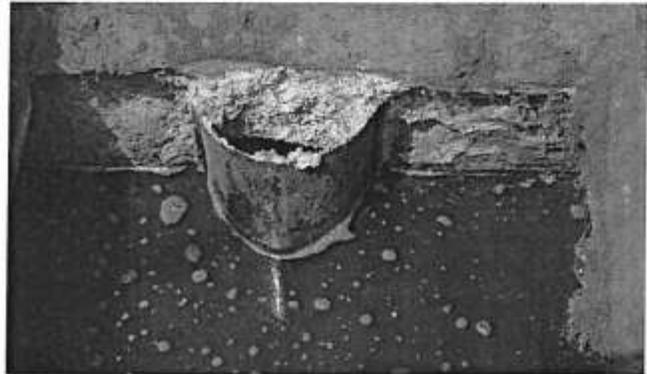
Illustration 1: Concrete Corrosion around Outlet Baffle
